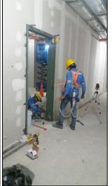
Depending on design, the frames are secured using metal straps.
