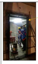
Timber strips at the other end during grouting of cement.
