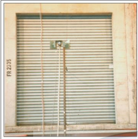
TACAM Shutter at START of 6 Hours Fire Test at Warrington Fire Research Centre (U.K.)
